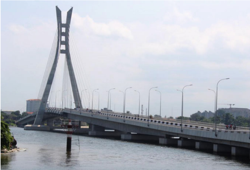
Fig. 28.5 Lekki-Ikoyi link bridge. Source [29]
