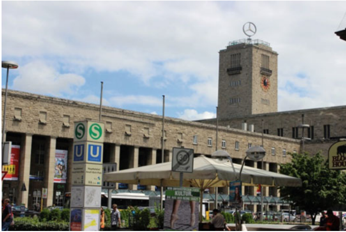
Fig. 11.11 Stuttgart Main Station
